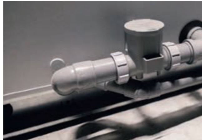
Balsifon: allows condensation water from the air handling unit directly into the sewer.
