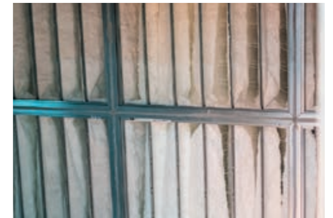
Air filters keep supply and return air clean. Ned Air offers a wide range of premium air filters. This means there is always a suitable solution for every specific application, such as filtering particulate matter.
